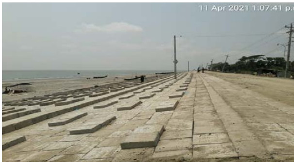
Figure 3-34: Slope Protection work from KM 30+800 to Km 31+450 in Polder-48
