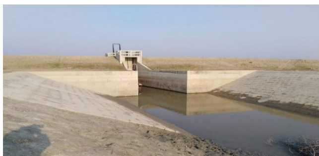
Figure 3-9: Completed DS of Polder-32
