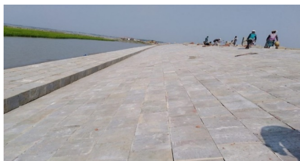
Figure 3-10: Completed Slope Protection Works in Polder-32
