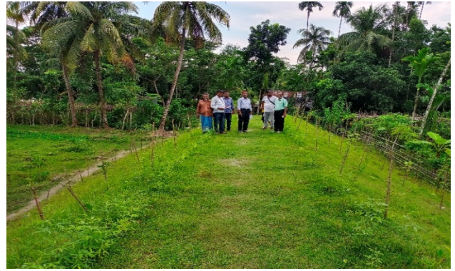
Figure 3-31: Embankment turfing and afforestation work at km 1+170 in Polder-39/2C
