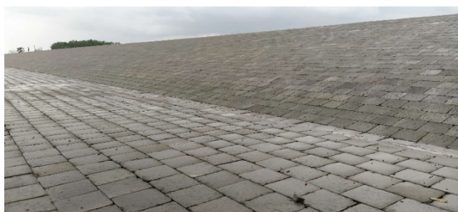
Figure 3-13: Nalian Closure Dam of Polder-32
