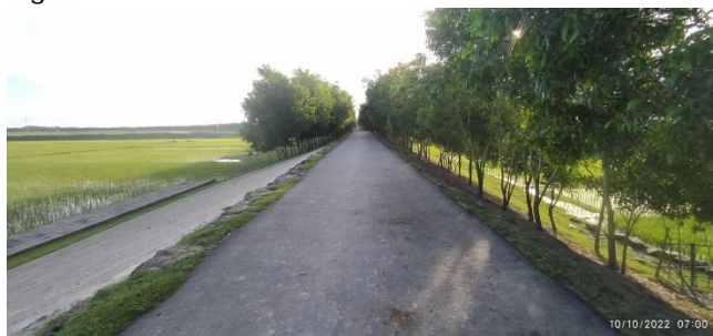
Figure 3-15: Completed Embankment of Polder-32
