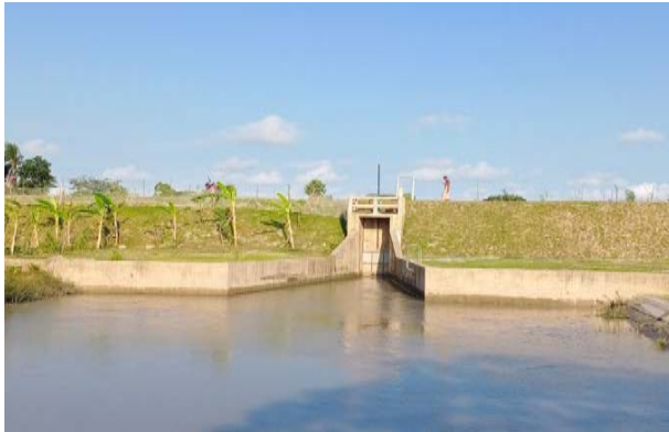
Figure 3-32: Complete Drainage Sluice DS-1 in Polder-40/2
