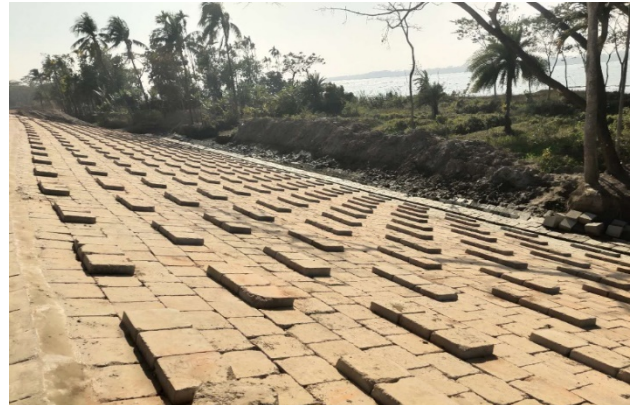
Figure 3-33: Slope Protection work For KM 48+672-48+764 in Polder-39/2C
