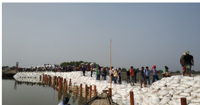
Figure 3-11: Nalian Closure Dam of Polder-32
